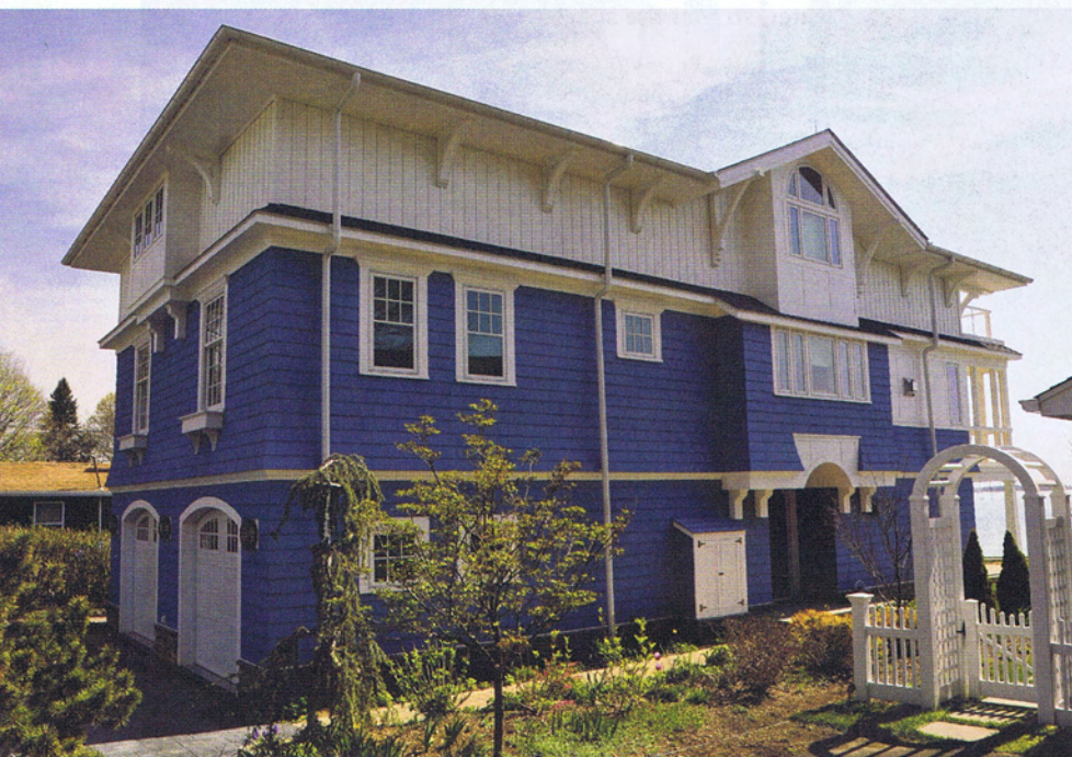
A variety of siding materials, such as New England shingle siding, board and batten and crown molding visually break up the boxy shape of the house.
