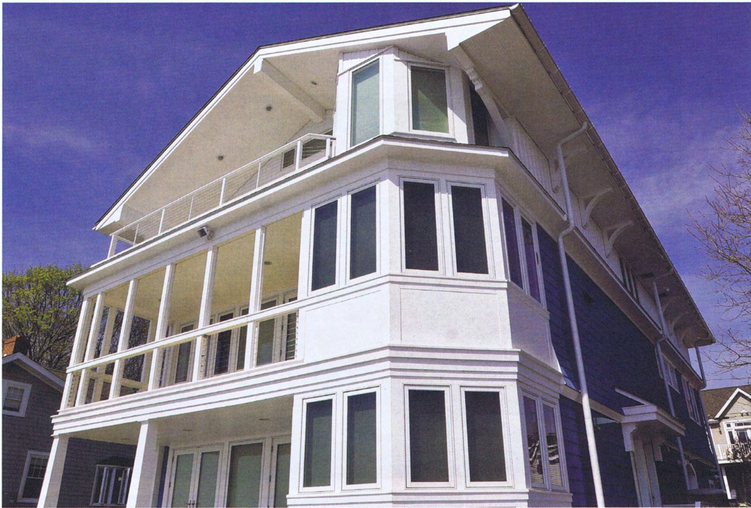
The roof shape may be simple, but the gable facing the water and decorative brackets lend depth and shape.
